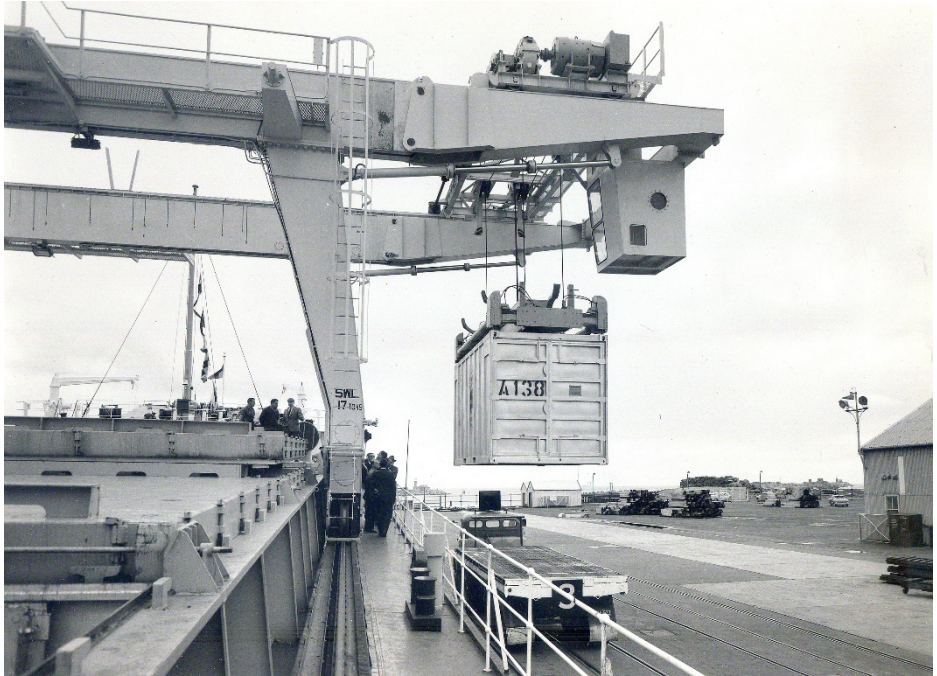
Image 20: Kooringa crane handling an Australian A container. Near the bottom centre of the image the crane rail and deck gear rack can be seen. Above the container the crane folding birdwings are extended over the wharf and the trolley has runout over them. The 6 ft to 8 ft extension corners on the spreader that caused trouble in Port Melbourne are easy to identify. The bottom birdwing pivot pins withdraw to allow the birdwing to fold down ready for sea and then a section of the birdwing acts as a stop to prevent trolley movement over the side.
