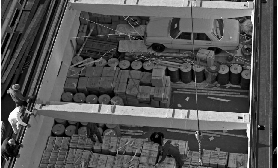
Images 2&3: Atrevida Fremantle harbour May 1968. Workers lashing break bulk cargo
