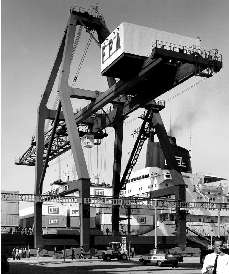
Image 30: The Fremantle Port twin lift StS crane working Encounter Bay outward bound on her maiden voyage. Twin 20 ft containers are suspended as they are discharging from deck cargo. The man in the bottom RH corner is the NZ born supervisor who recognised the Meckering earthquake for what it was and ran to the wharf to check on the Hoskins commissioning team.
